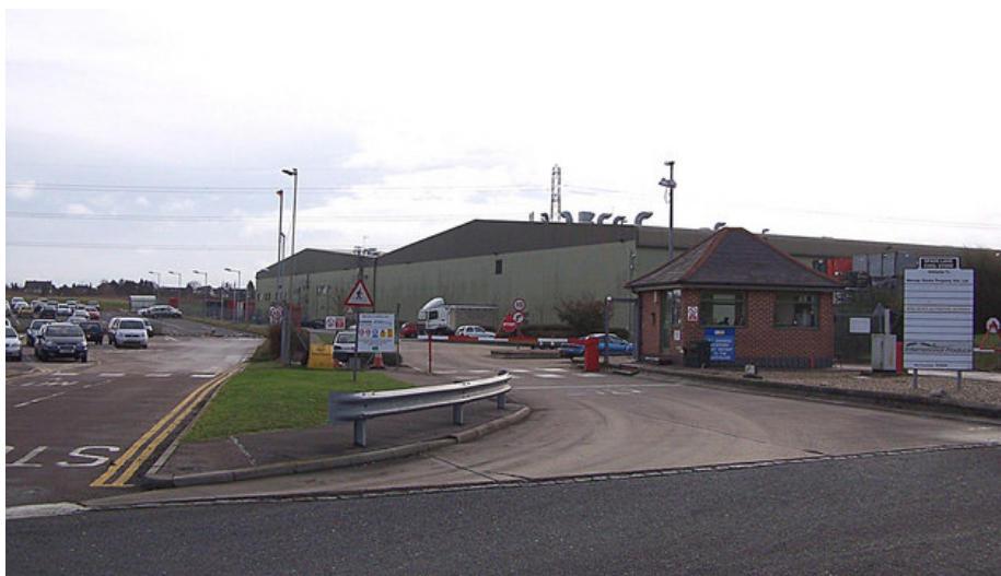
Spade Lane Cold Store built about 30 years and subsequently virtually destroyed in a huge fire. Now fully rebuilt, and largely used by International Produce - a dedicated supply partner to ASDA, the UK's second largest retailer. Credit: Richard Dorrell.
