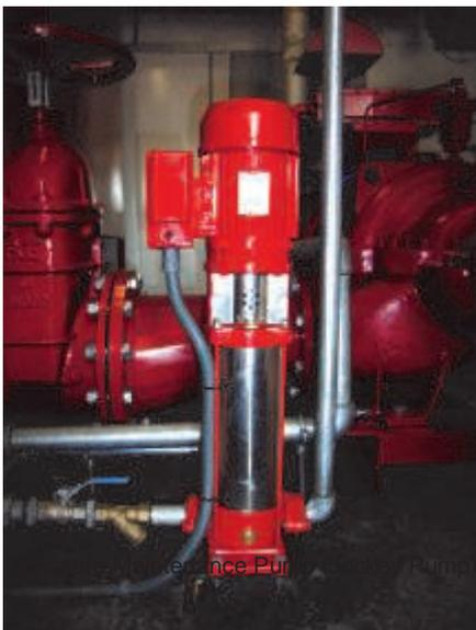
would stop and start in response to signals from a pressure switch mounted in the installation trunk main. The duty of the unit is small so that in the event of serious pressure loss the main fire pump would immediately be brought into operation.
