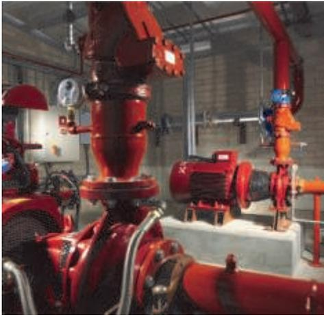
Two end suction electrically and diesel driven pumps
