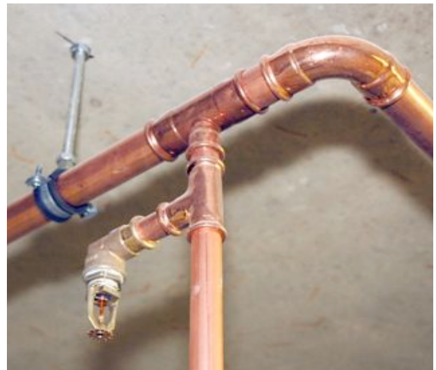
Fig. 10. Examples of low pressure watermist pipes and fittings.
