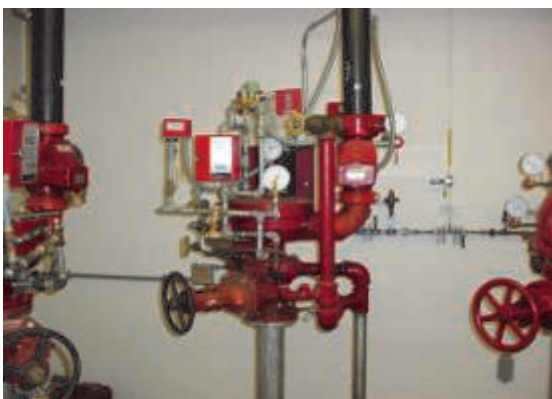
PREACTION type control valve
